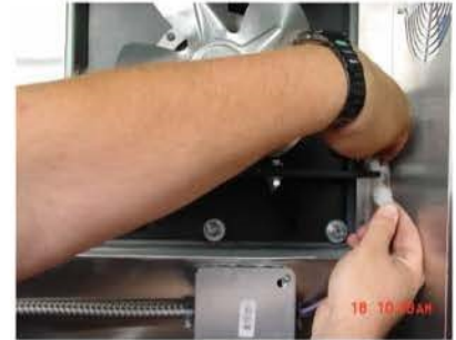
Step 3 - Unplug the Quick Disconnect.
