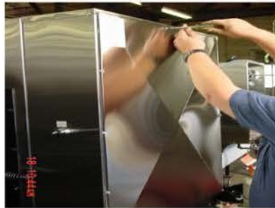
Step 2 - Remove Service Panel Located at the Back of the Unit.
